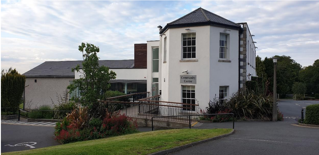
Photo 8: Mount Merrion Community Centre.
