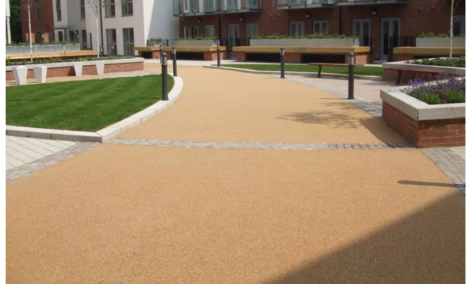
Fig 21 – Coloured Asphalt Surface
